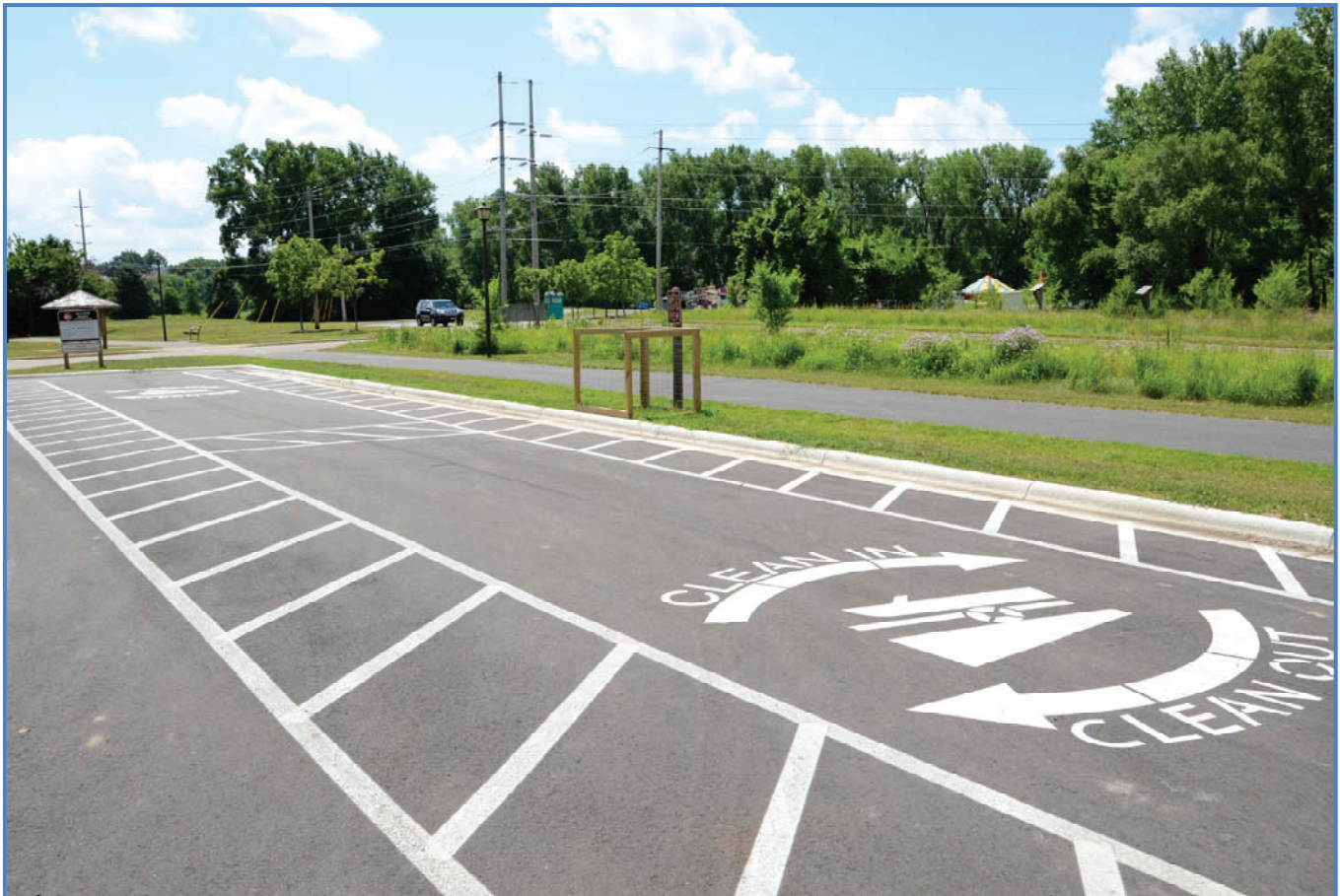
A clean drain and dry area with sign, disposal bin, and pavement stencil/parking box (MN)
